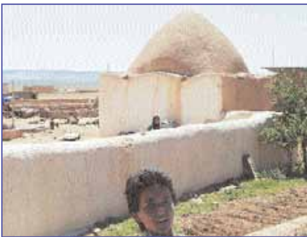
Rooftop water-harvesting system providing drinking and supplemental irrigation water in remote areas.
