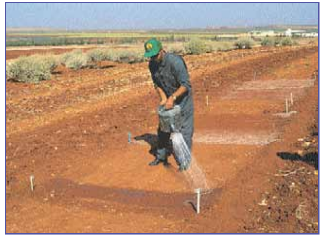
Emulsified paraffin wax developed in Iraq being sprayed on a micro-catchment to induce runoff near Aleppo, Syria.
