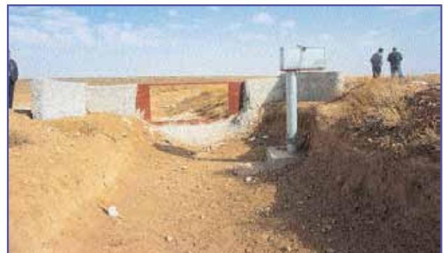
Low cost weirs may be installed on wadis to measure runoff rate from macro-catchments. This one is in Mouaaqar, Jordan.
