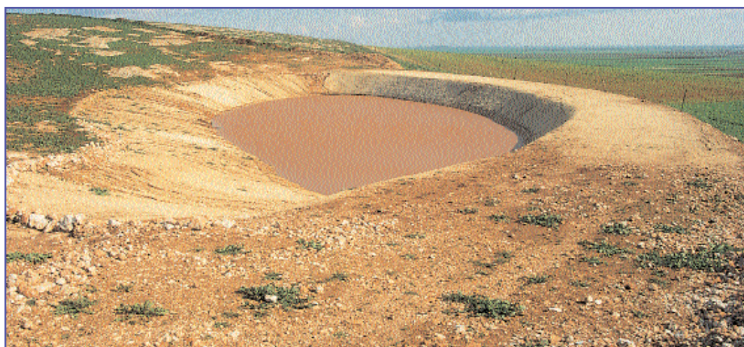
Small farm water-harvesting reservoir for supplemental irrigation of field crops at ICARDA research station in northern Syria.
