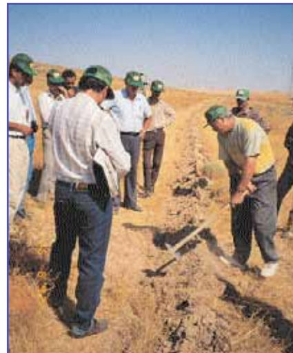
Proper construction of water harvesting systems requires skilled labor. Enhancing the capacity of people involved is usually needed.
