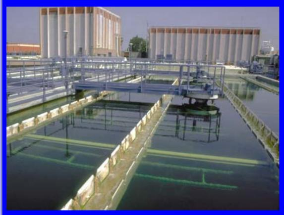
Microfiltration, reverse osmosis and UV/H<sub>2</sub>O<sub>2</sub> treatment for 250,000tpd of sewage works effluent for groundwater recharge commissioned 2007
