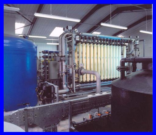
The membrane plant at Anglian Water's Flag Fen Sewage Treatment Works, commissioned 2001, treats 1,200tpd of final effluent for recycling as boiler make-up water in the adjacent power station
